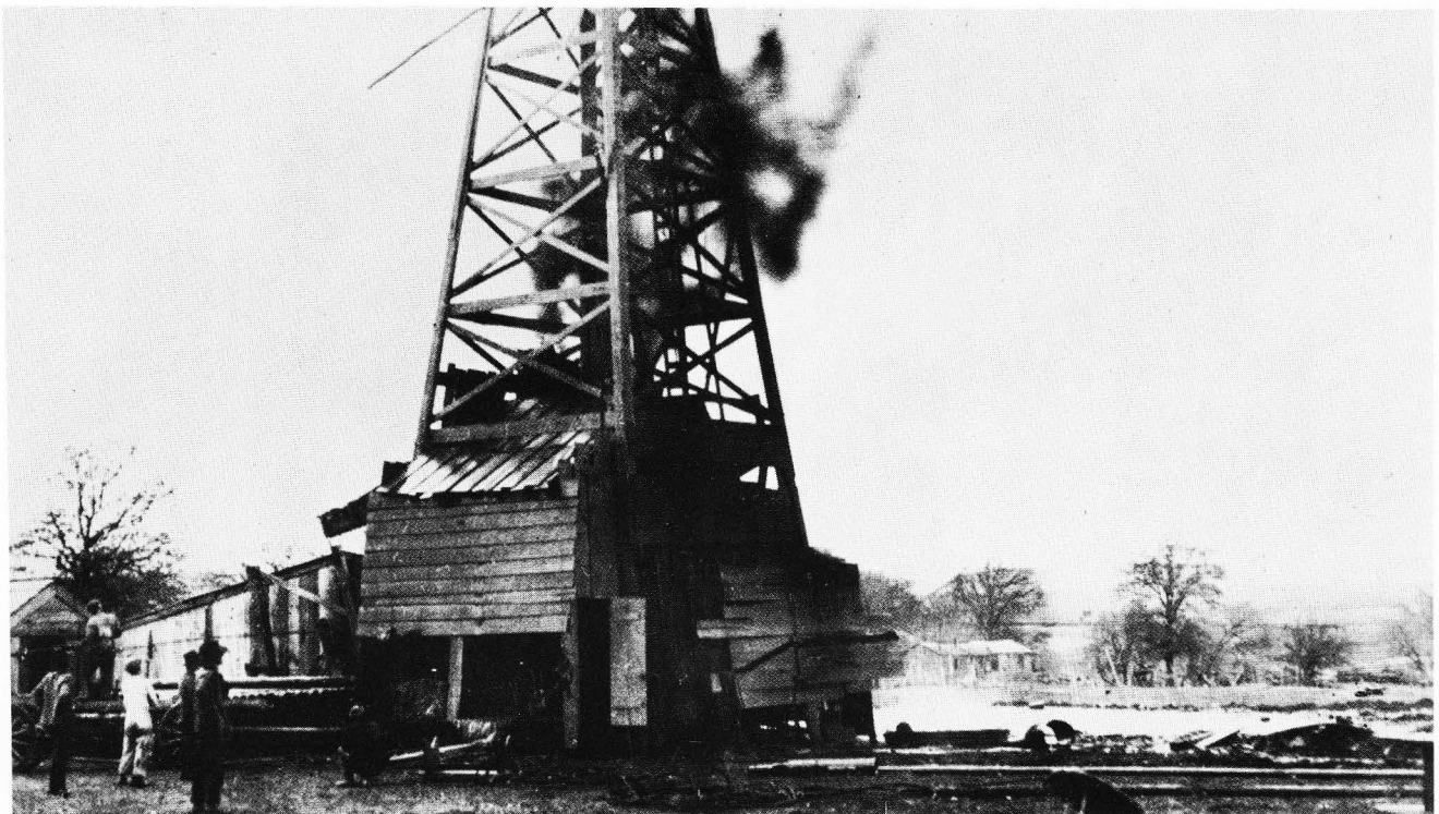
The Nora Brown. This was the first well brought in by the Gilcrease Oil Company.
